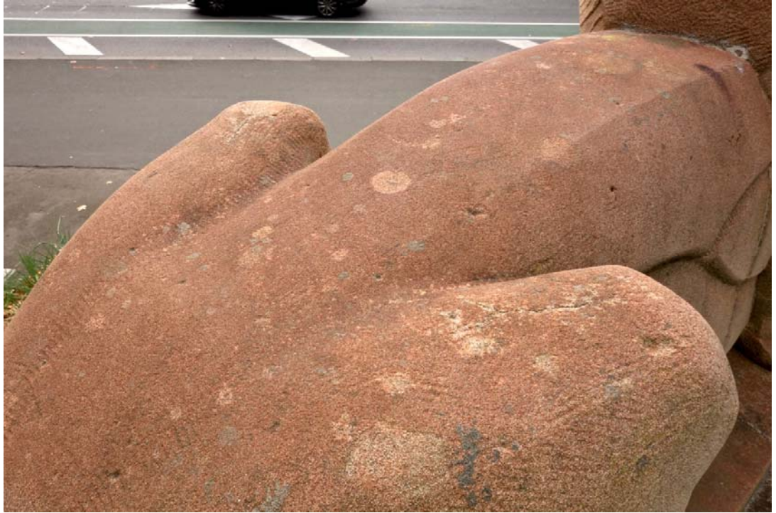
Figure 19. Back and hind-quarters of the eastern lion showing vertical cracks towards the knees in both legs and a spotted appearance due to growth of microflora, particularly lichens. Previous removal of the lichens (in 2009) has left shallow 'craters' in the surface of the stone, such as the one in the centre of the image. The iron-stained case-hardened surface of the stone has been lost from these 'craters', risking increased rates of stone decay.
