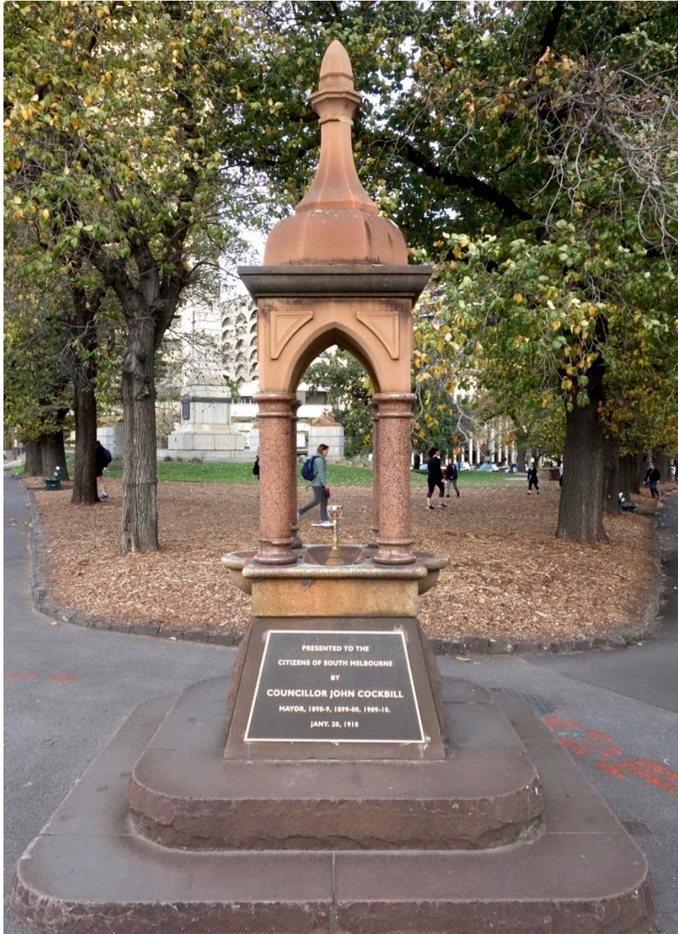
Figure 20. Drinking fountain showing some small losses of moulding details, and iron and biological staining of stonework. In the background, note pedestrian traffic across the tan-barked northern corner of the Reserve (see section 2.3.2).
