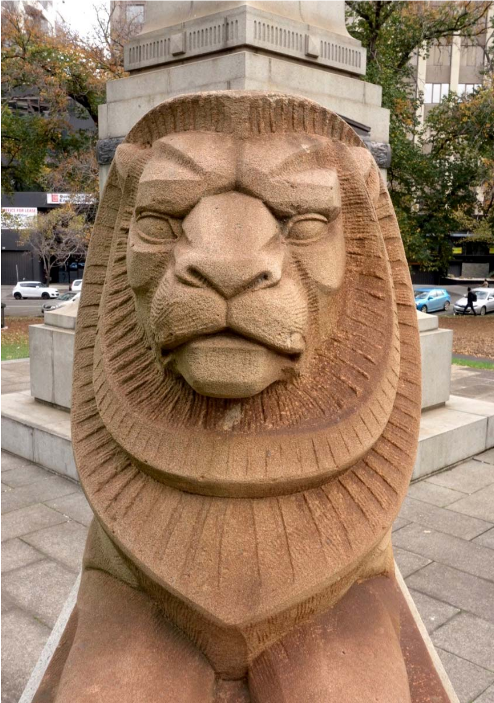
Figure 18. Eastern lion showing strong iron-oxide staining on the right (northern) side closest to the St Kilda Road trams. In contrast, the left (southern) side has little rust staining and some green algae, as it faces the prevailing weather.
