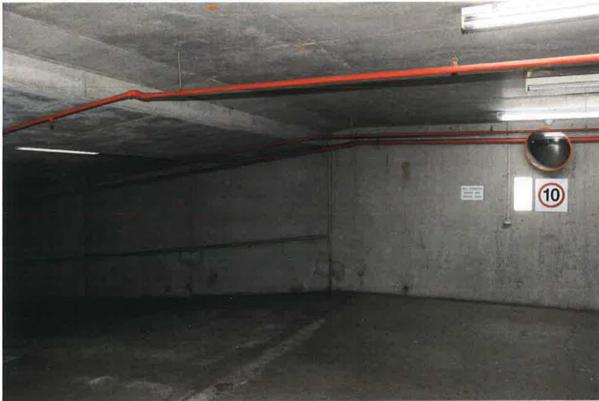
05 - Ramp B1 - Lower Ground
