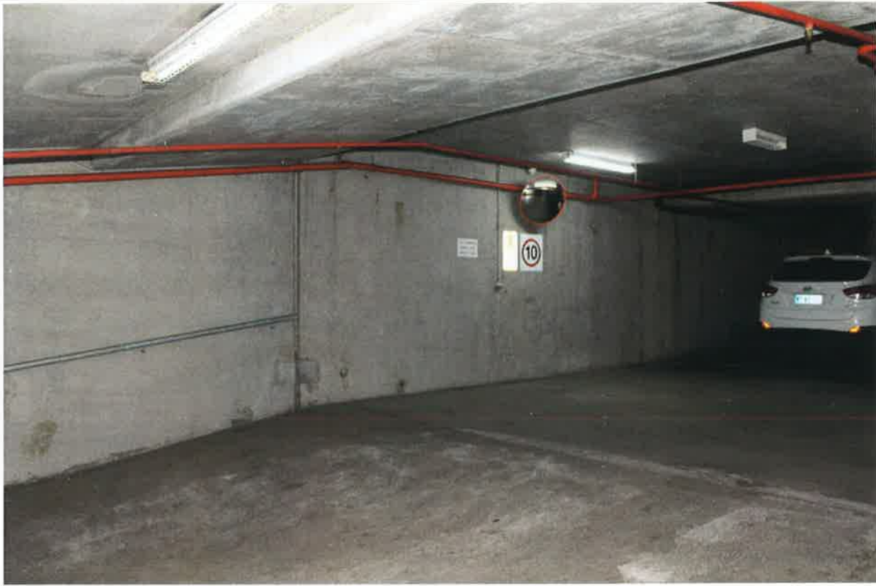
04 - Ramp B1 - Lower Ground
