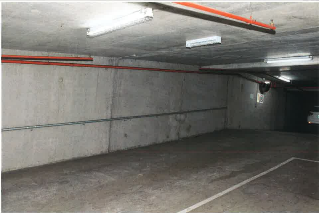
02 - Ramp B1 - Lower Ground
