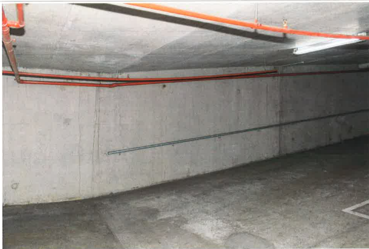
01 - Ramp B1 - Lower Ground
