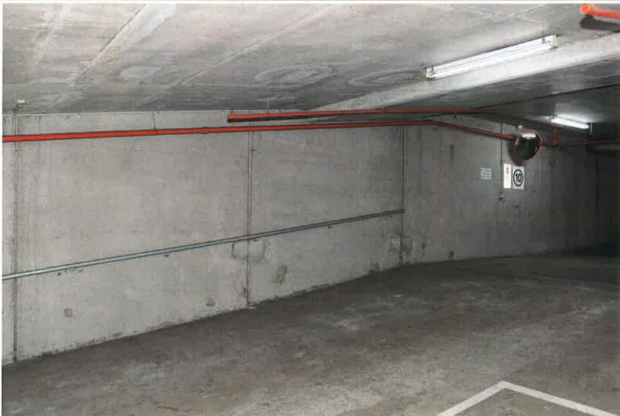
03 - Ramp B1 - Lower Ground
