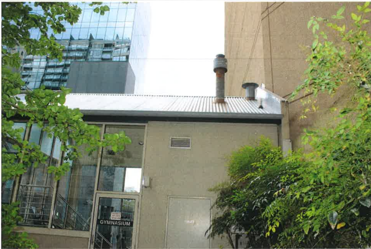
24 - East Facade - Pool Building
