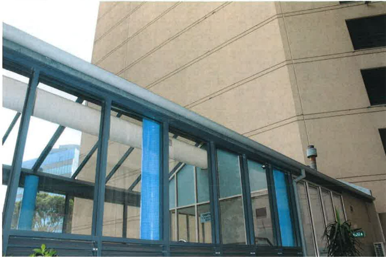
17 - East Facade - Pool Building
