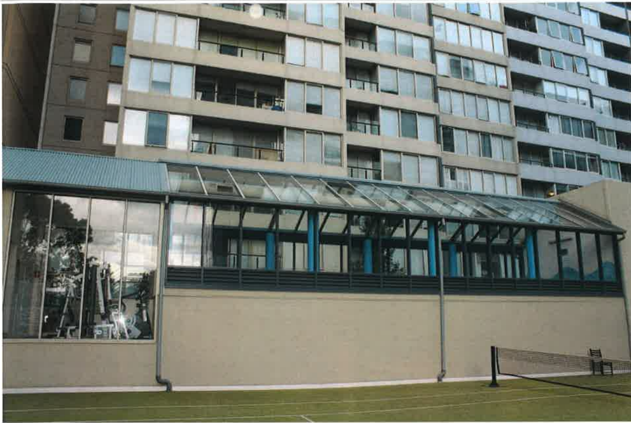
02 - West Facade - Pool Building
