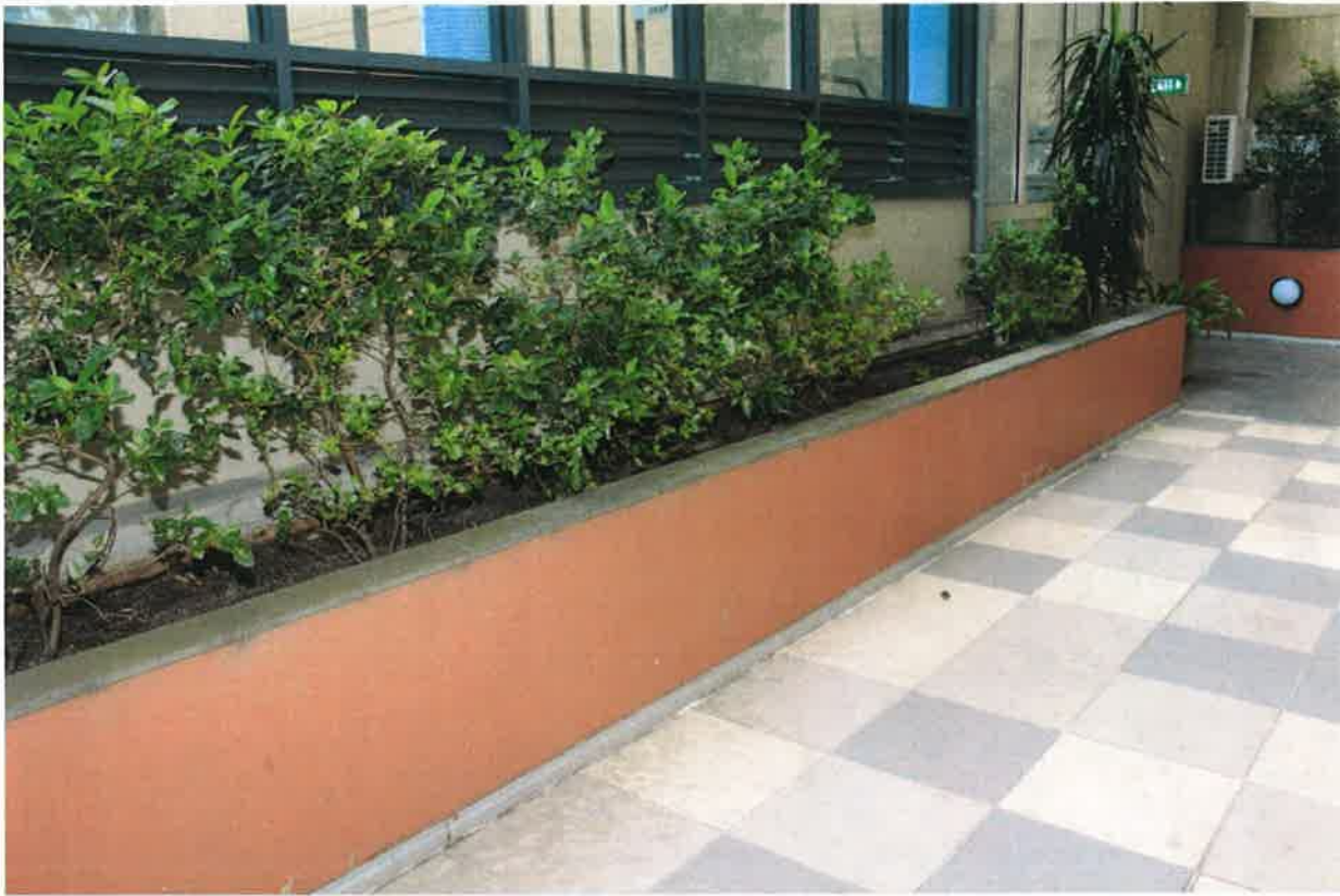
15 - East Facade - Pool Building
