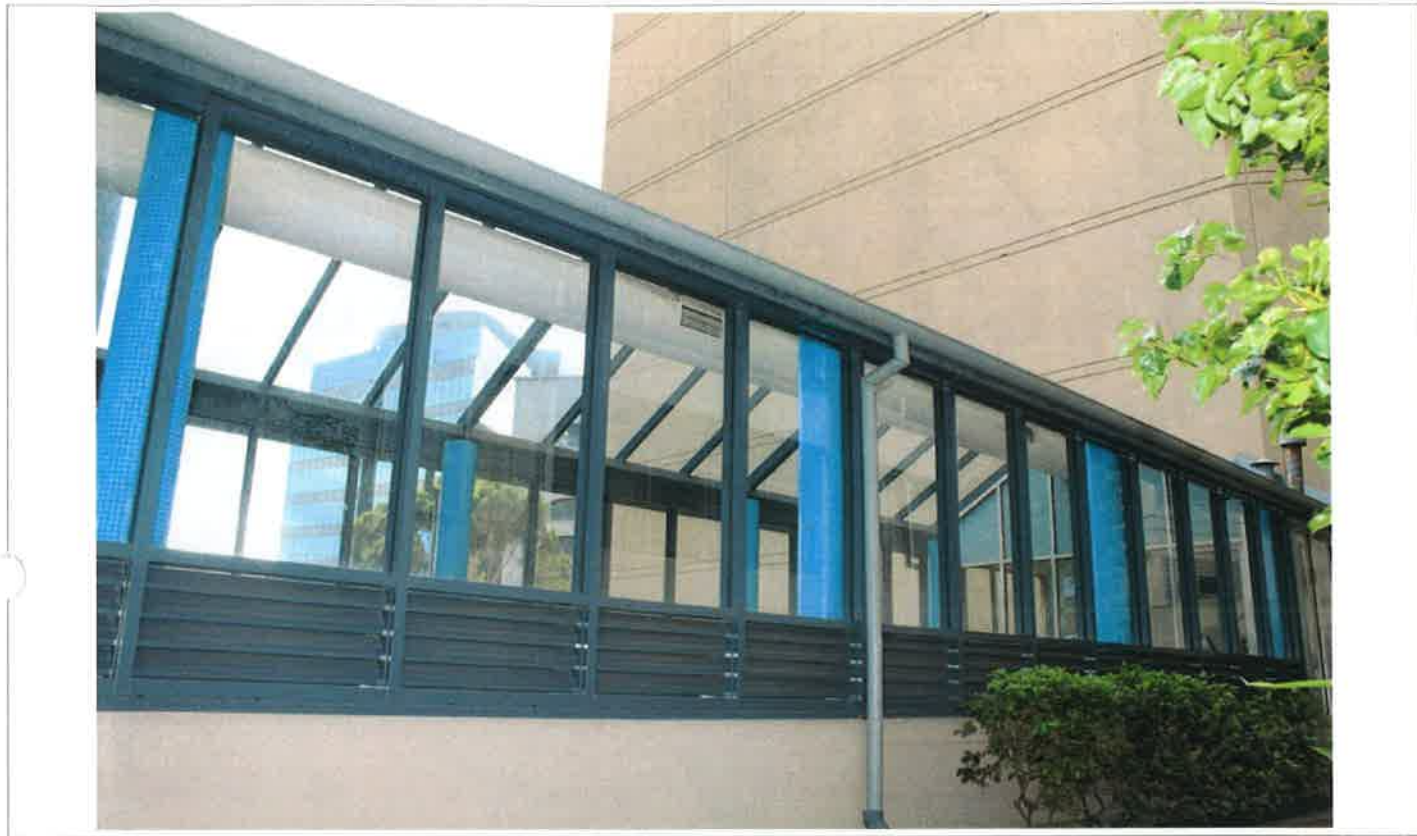
11 - East Facade - Pool Building
