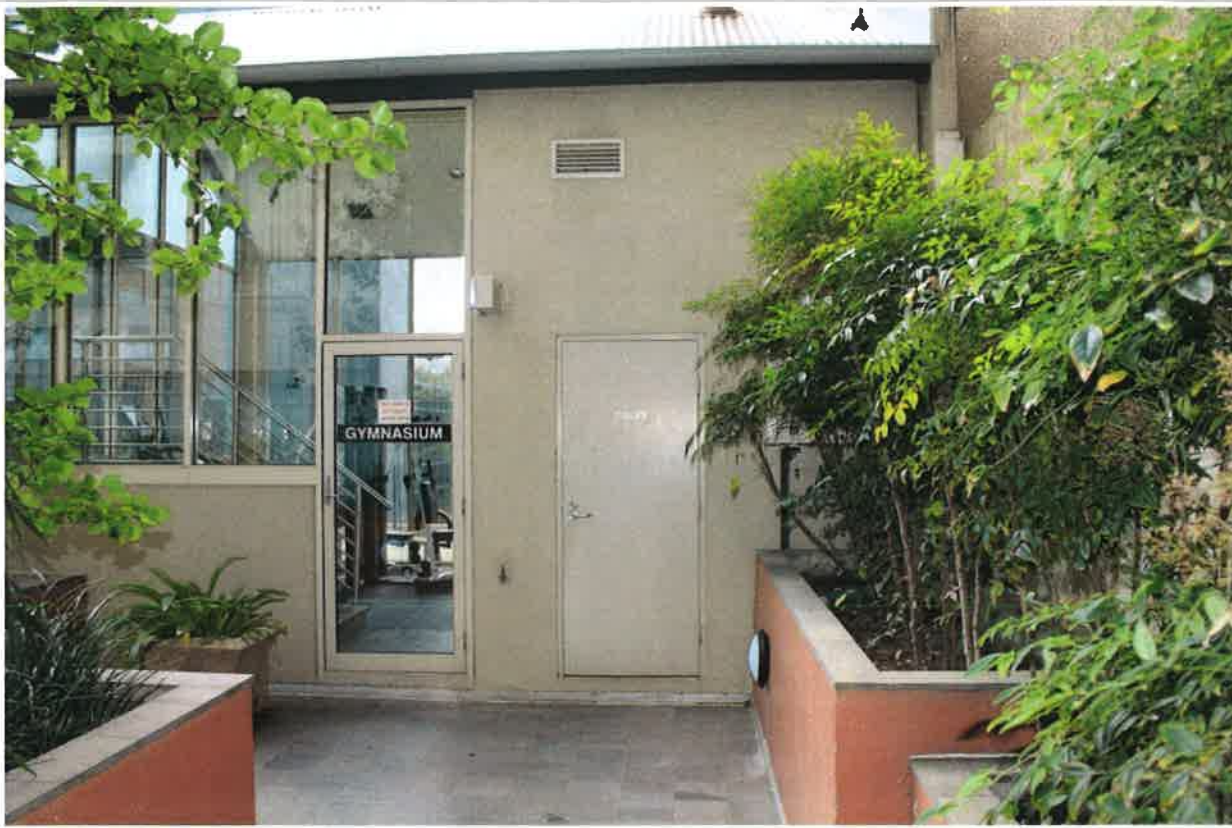
23 - East Facade - Pool Building
