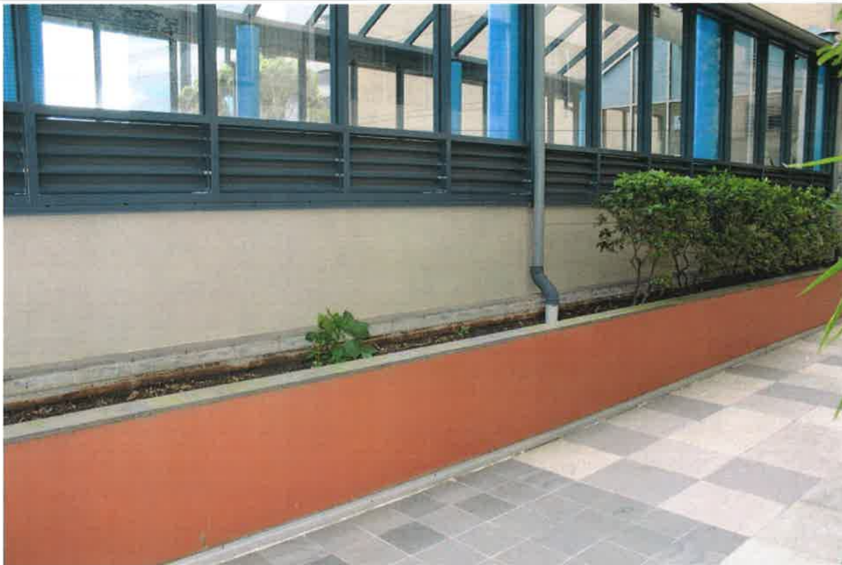
10 - East Facade - Pool Building
