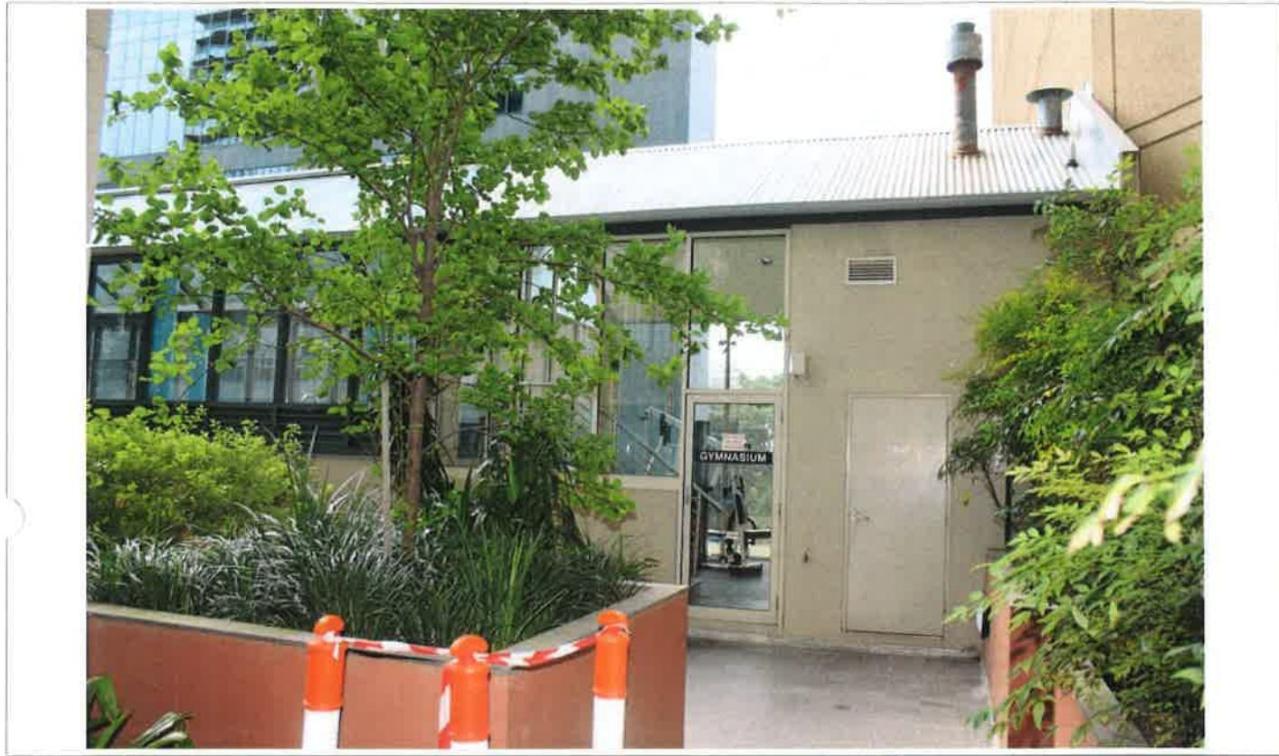
27 - East Facade - Pool Building
