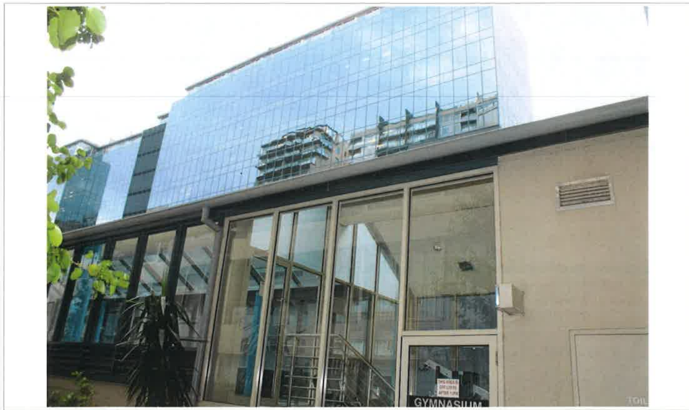
22 - East Facade - Pool Building
