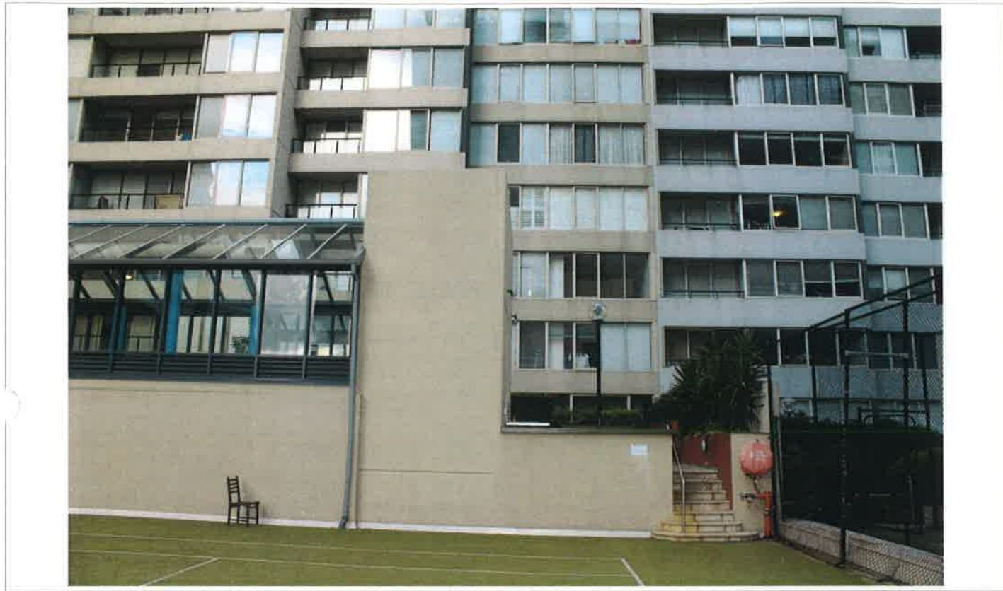
04 - West Facade - Pool Building
