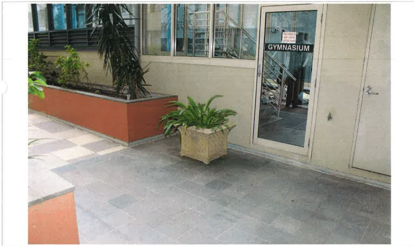
20 - East Facade - Pool Building
