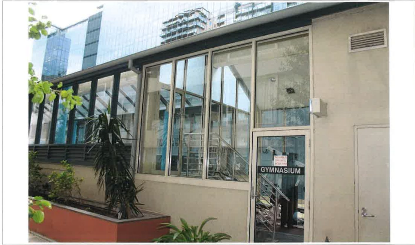
21 - East Facade - Pool Building
