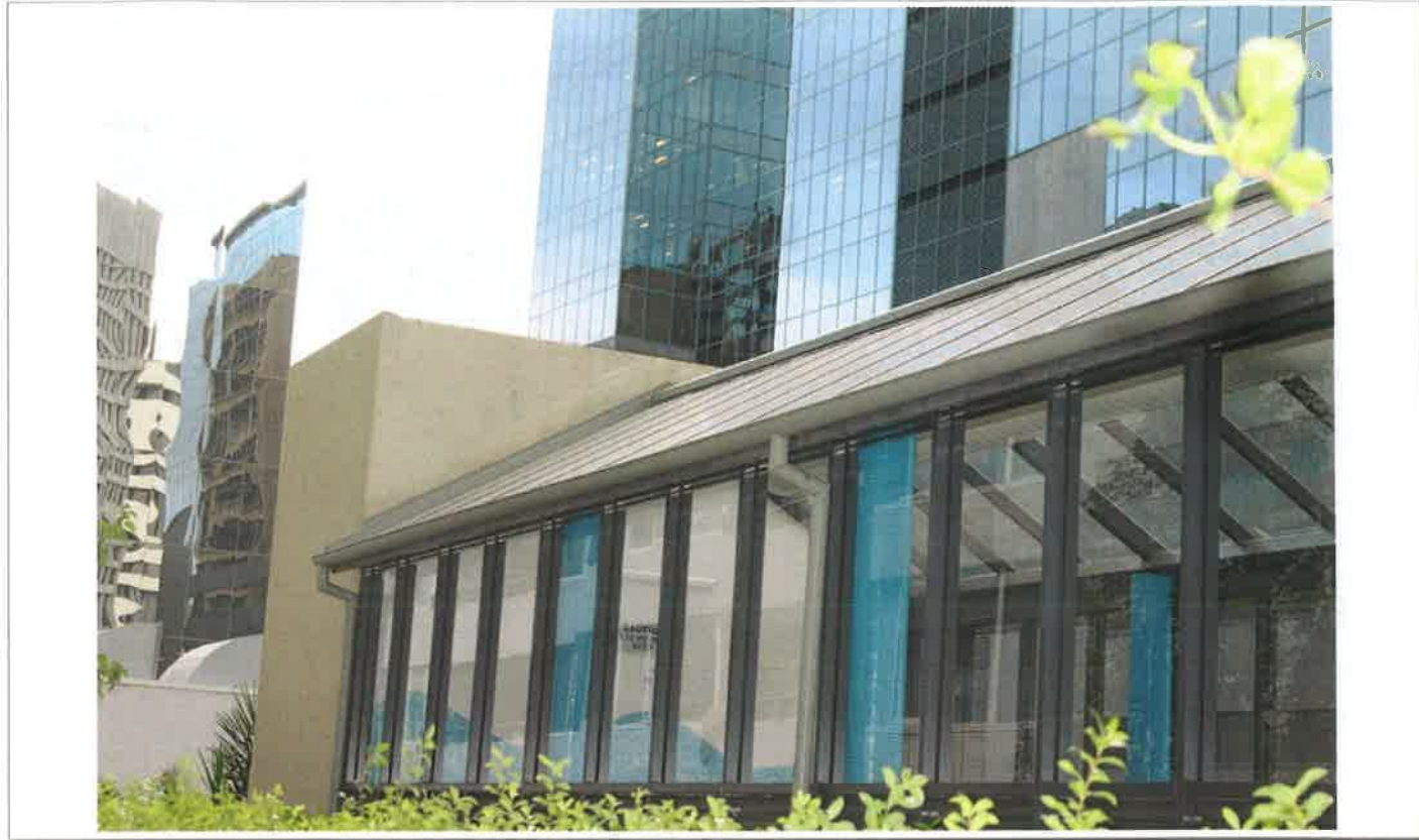
25 - East Facade - Pool Building
