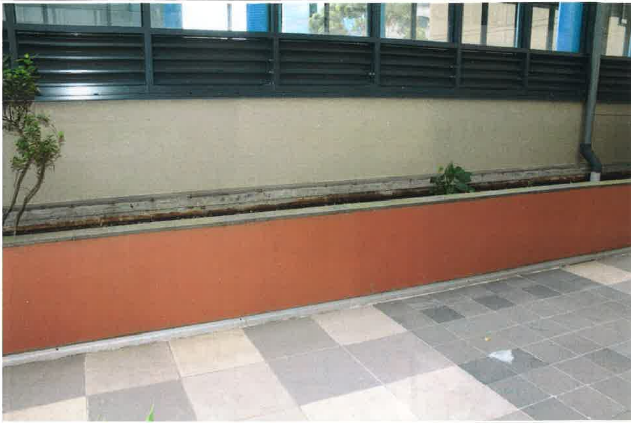
07 - East Facade - Pool Building
