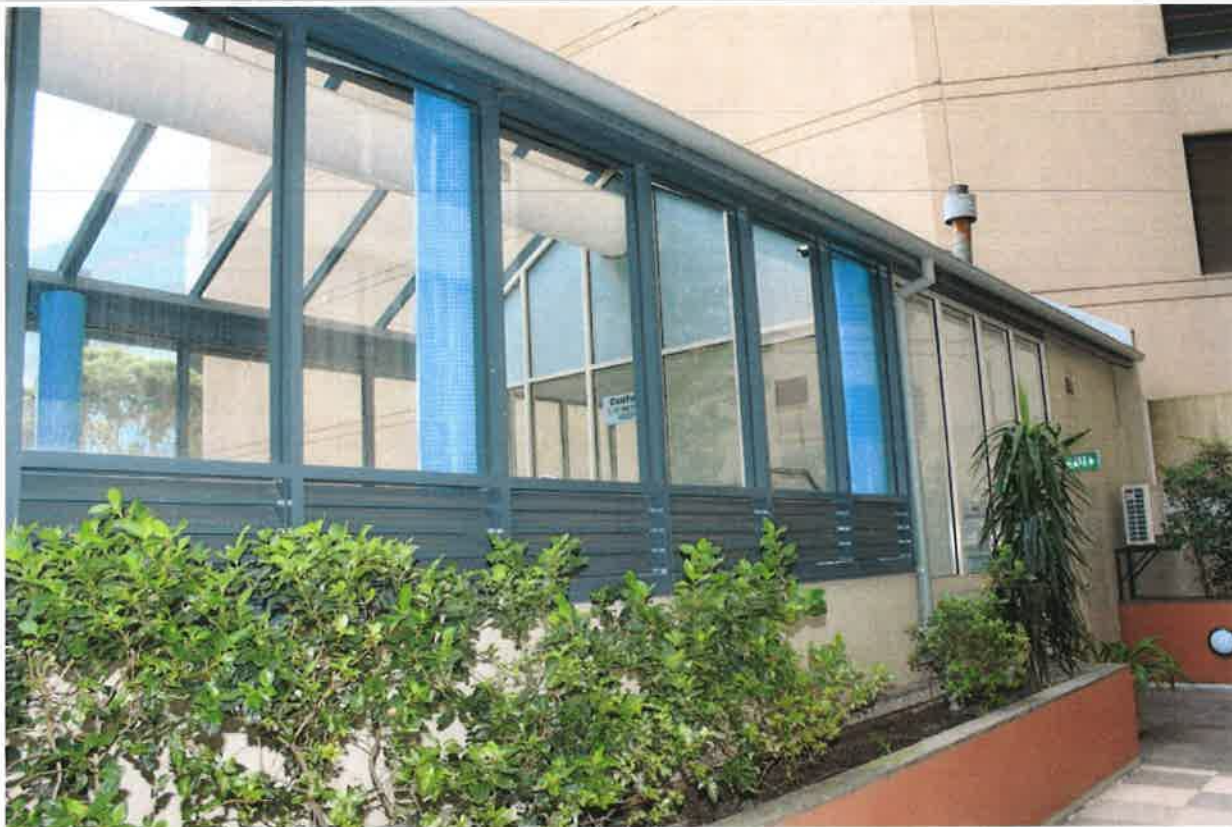
16 - East Facade - Pool Building
