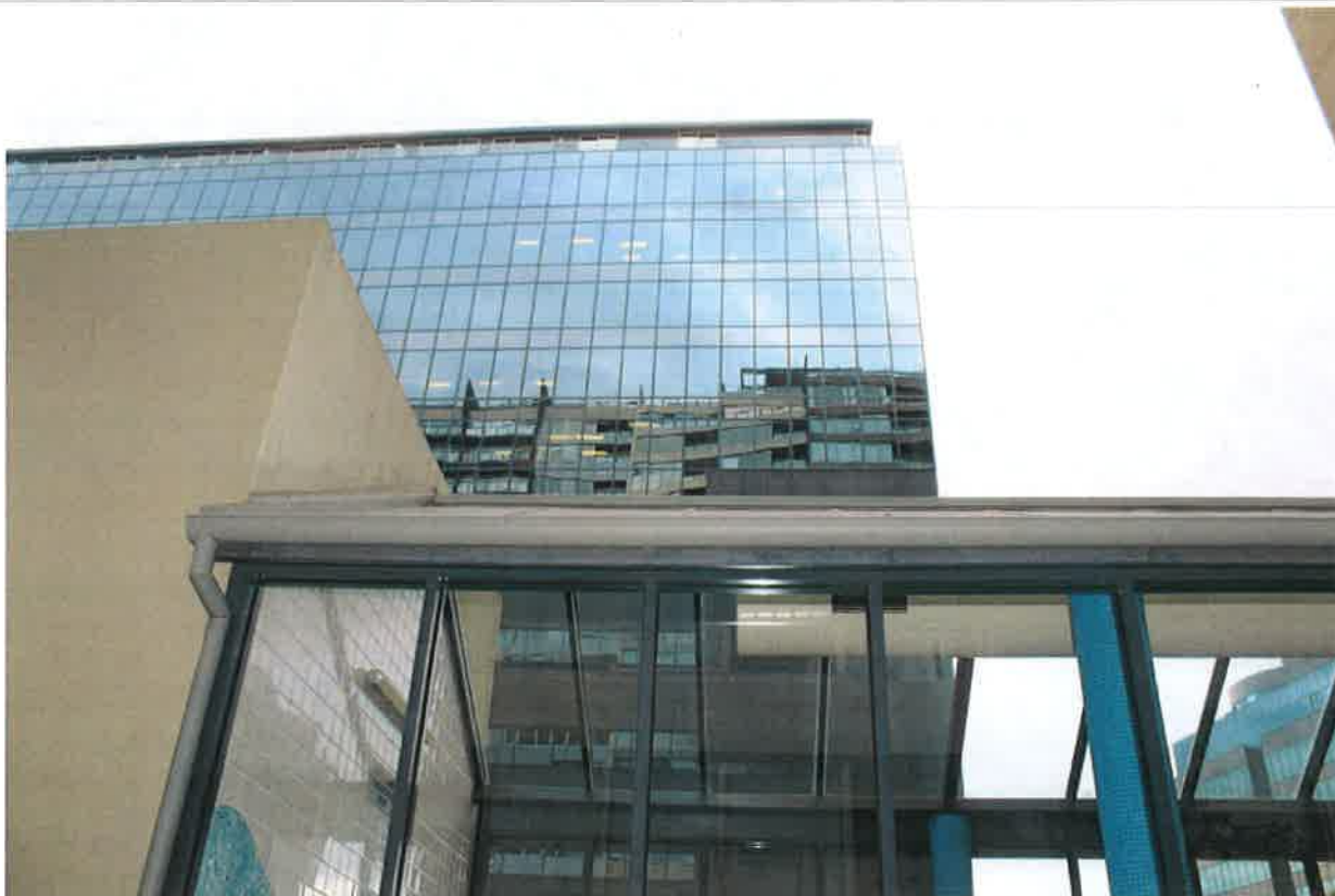
06 - East Facade - Pool Building
