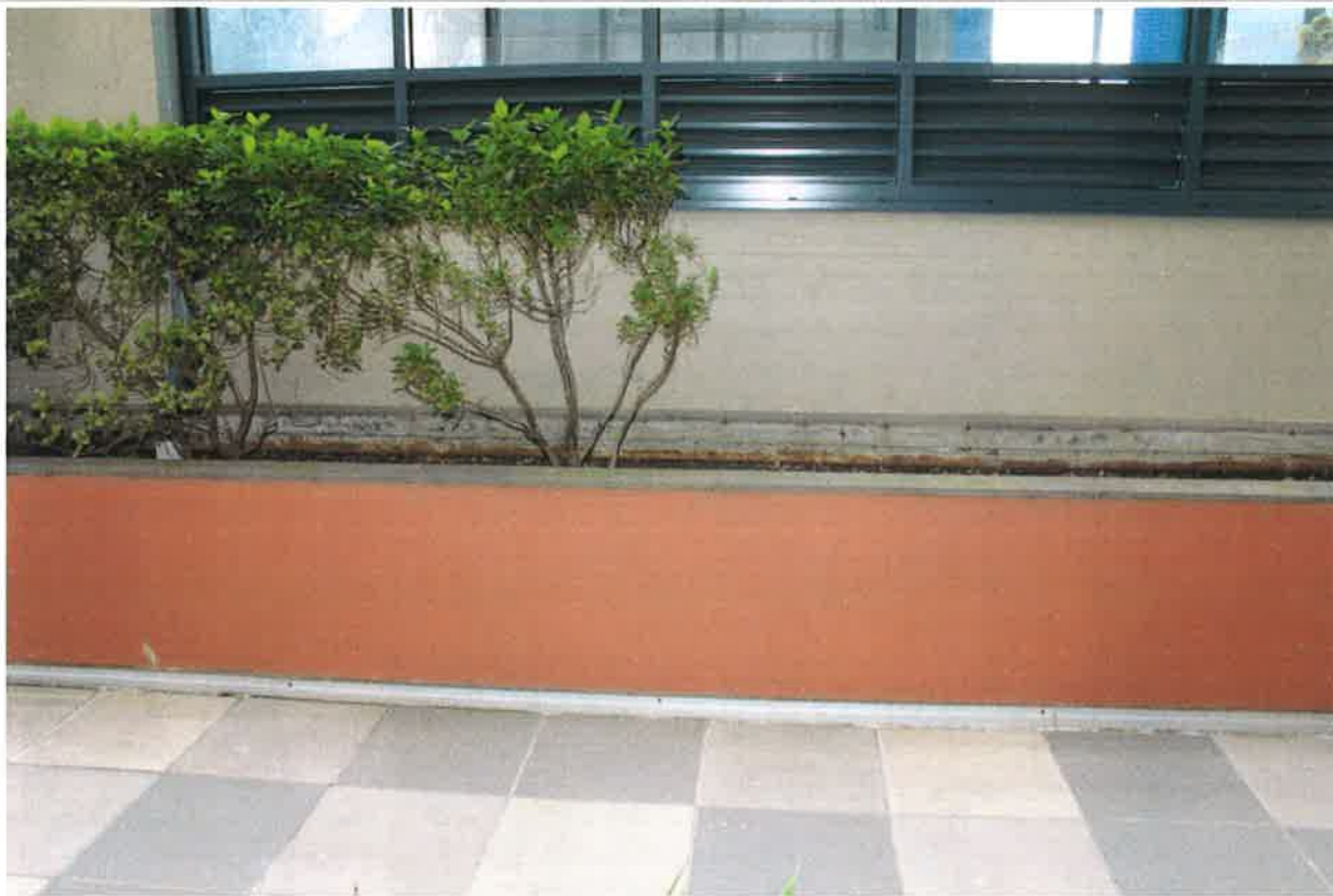
04 - East Facade - Pool Building
