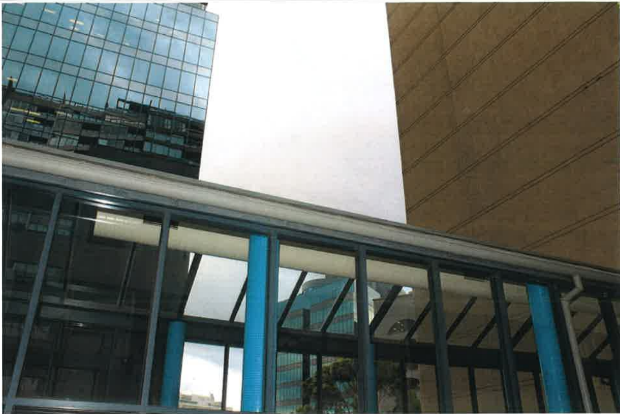
09 - East Facade - Pool Building
