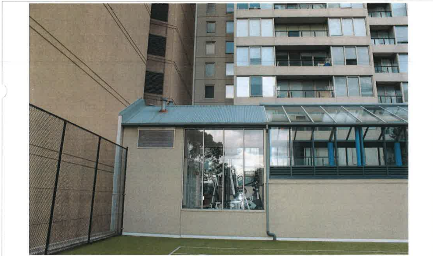
01 - West Facade - Pool Building
