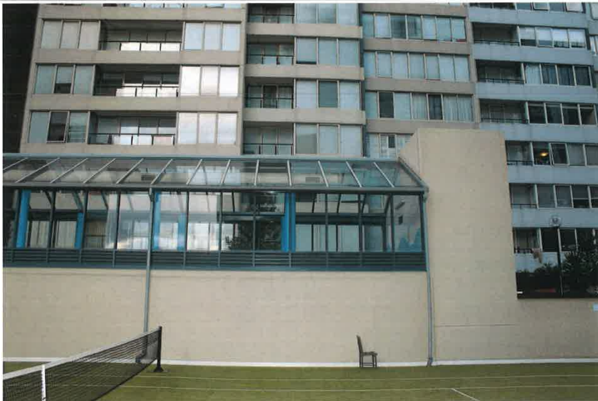
03 - West Facade - Pool Building
