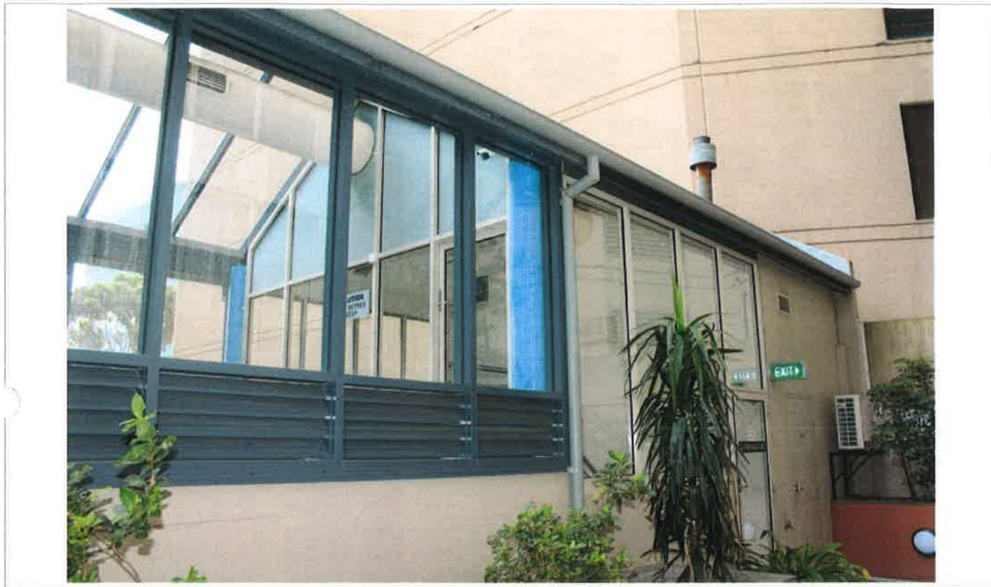
19 - East Facade - Pool Building
