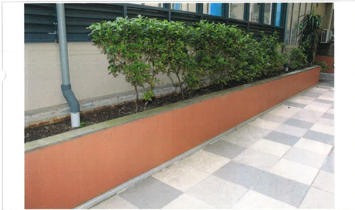
12 - East Facade - Pool Building
