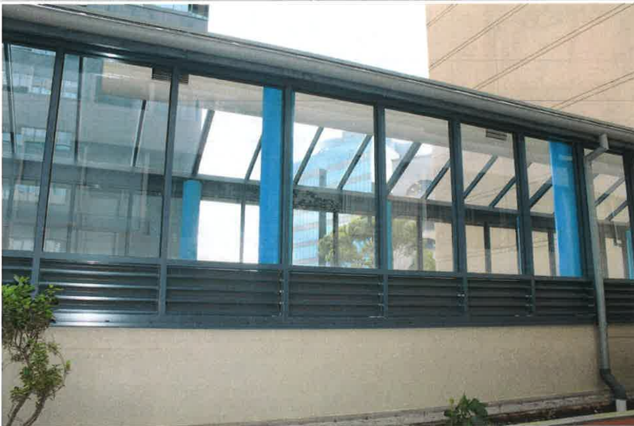
08 - East Facade - Pool Building
