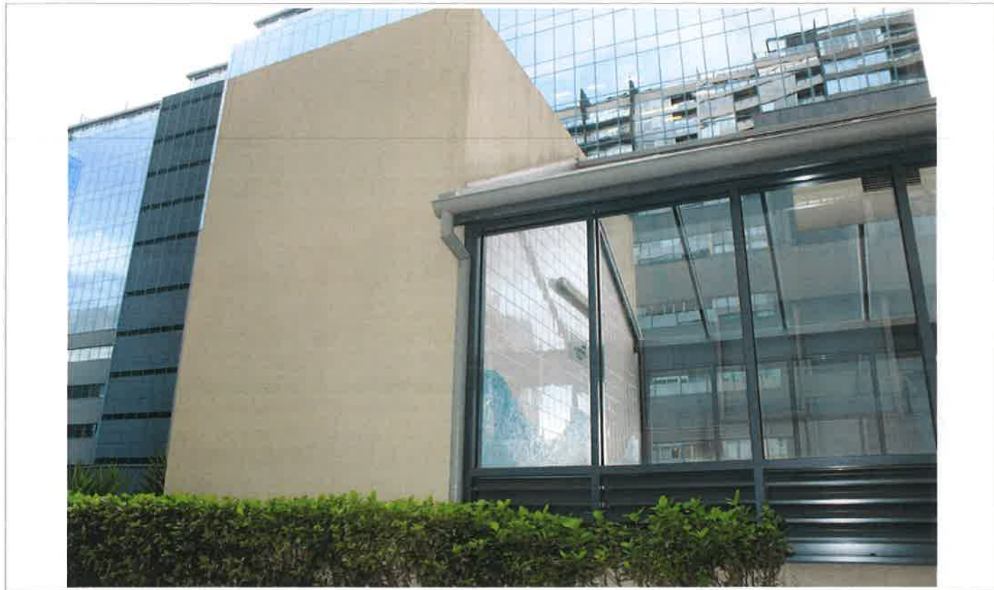
02 - East Facade - Pool Building
