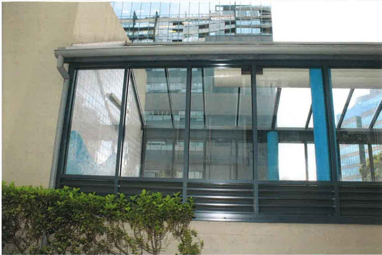
05 - East Facade - Pool Building
