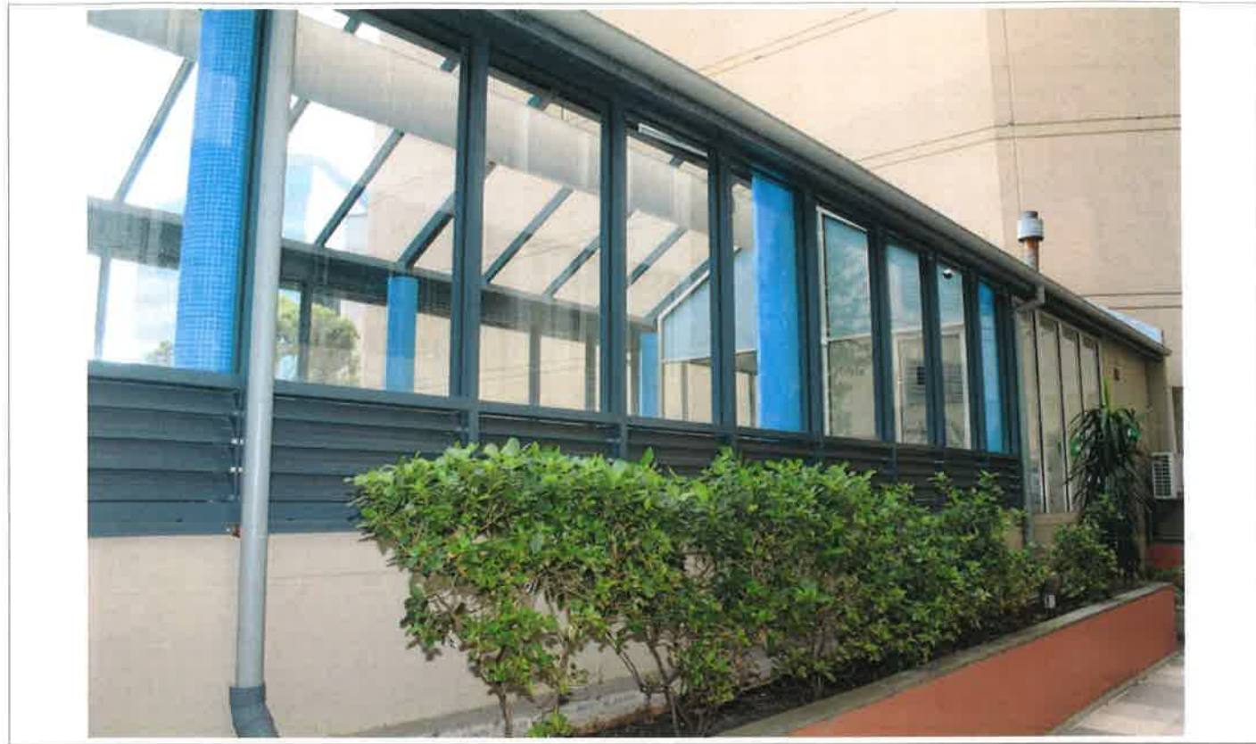
13 - East Facade - Pool Building
