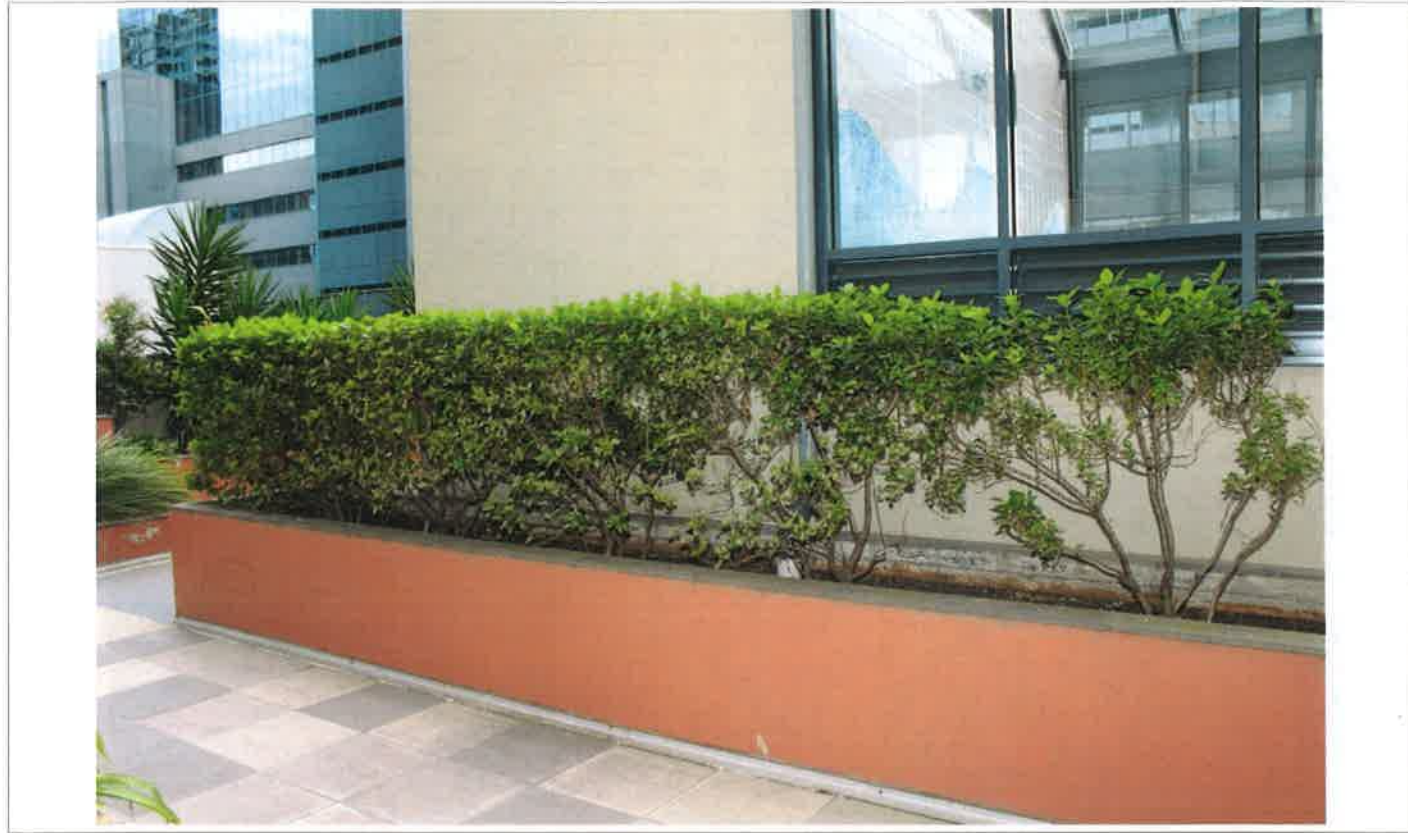
01 - East Facade - Pool Building
