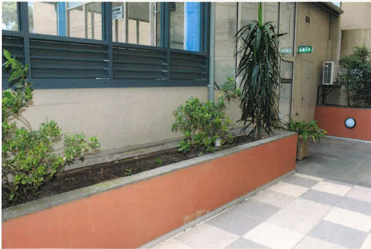
18 - East Facade - Pool Building
