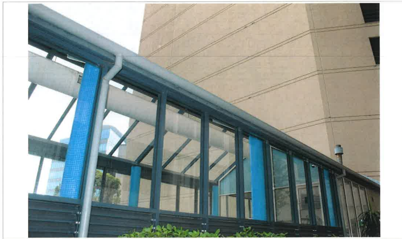
14 - East Facade - Pool Building
