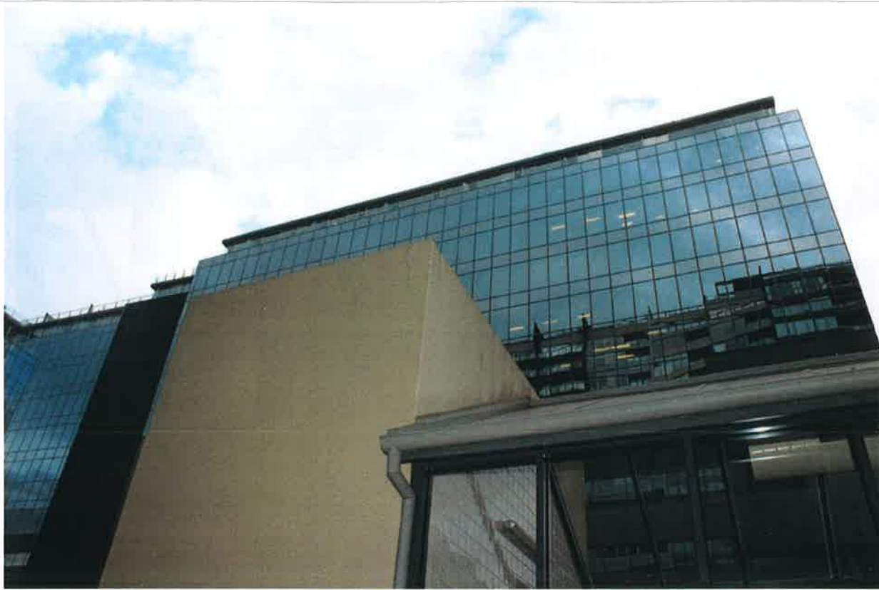
03 - East Facade - Pool Building
