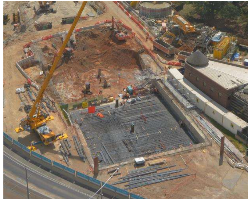
Staged roof construction in North box
