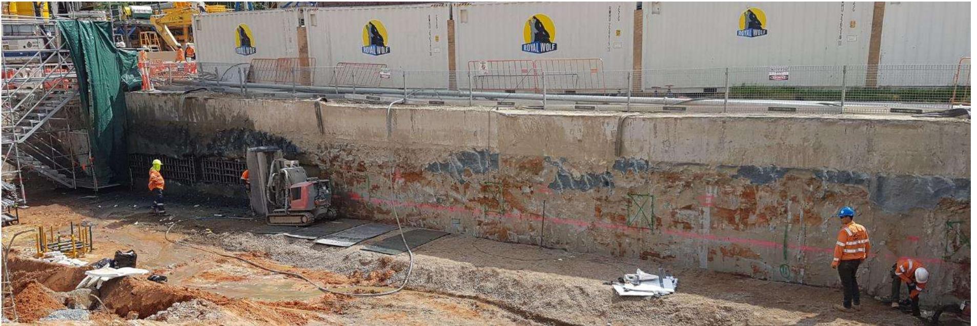
Aqua cutter robot works along the north box wall
