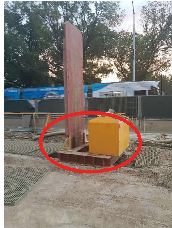
Stop end clamp in place
