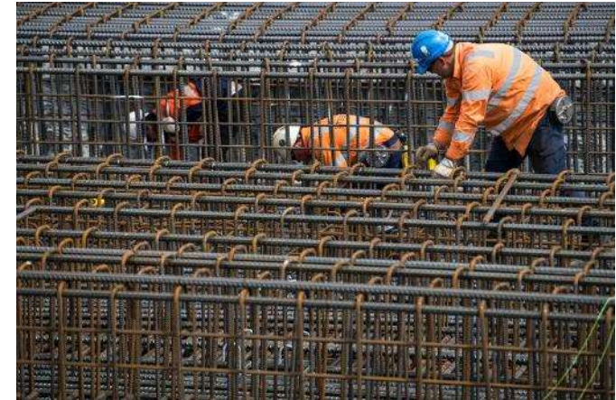
Steel tying works in the north box
