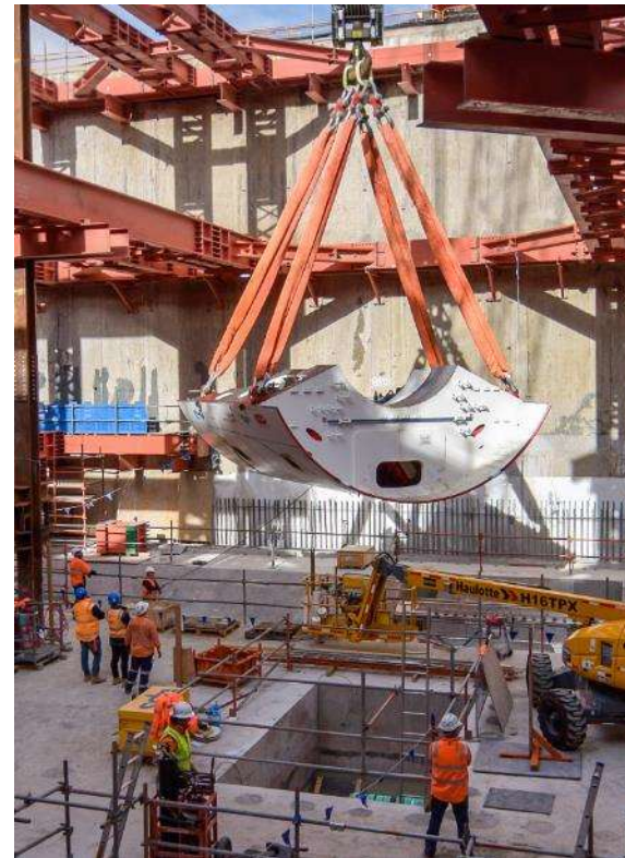
TBM parts lowered into place in the western section
