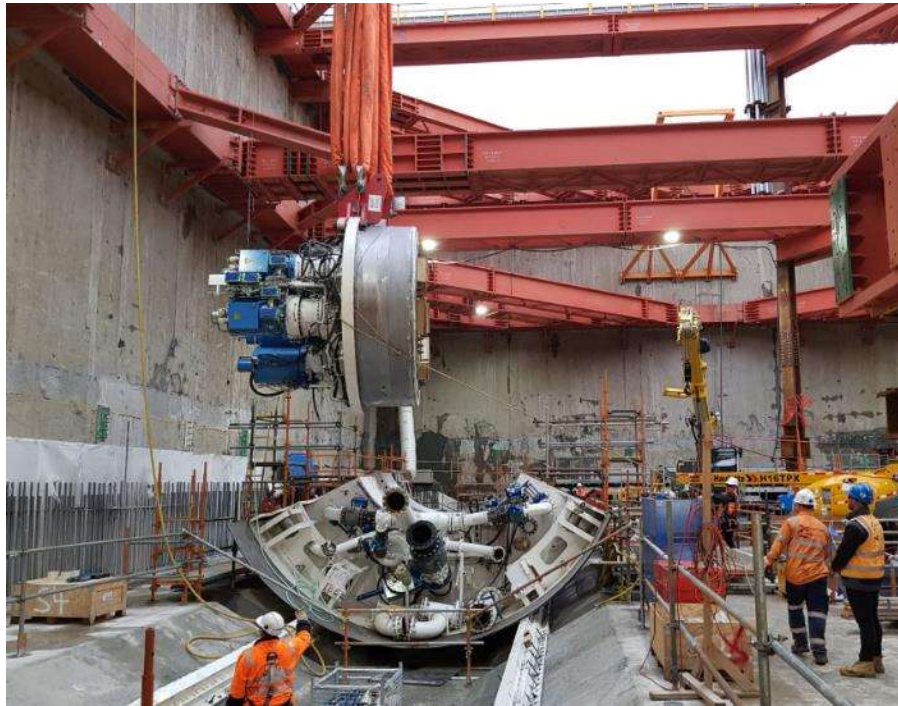
TBM parts lowered into place in the western section
