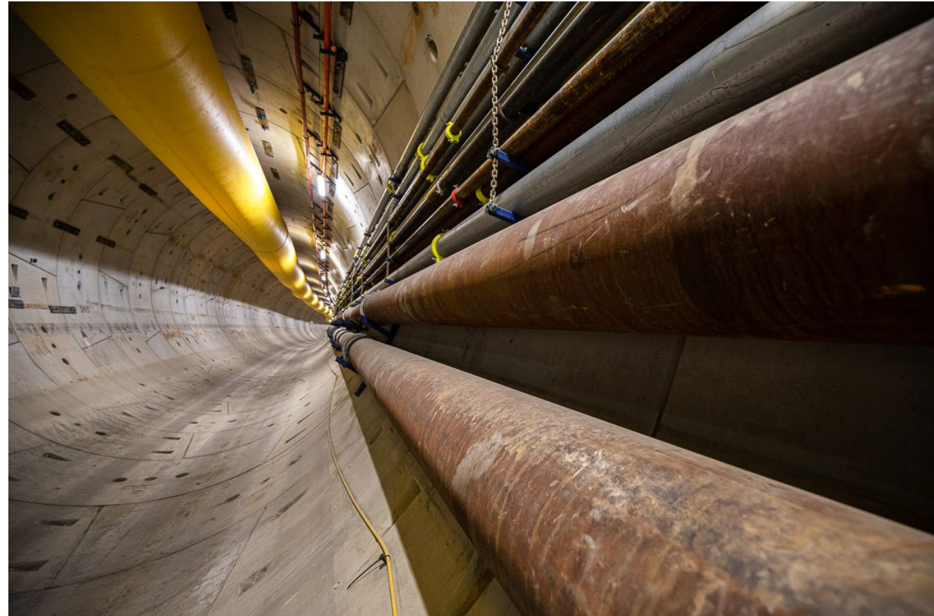
Pipes transporting excavated material
