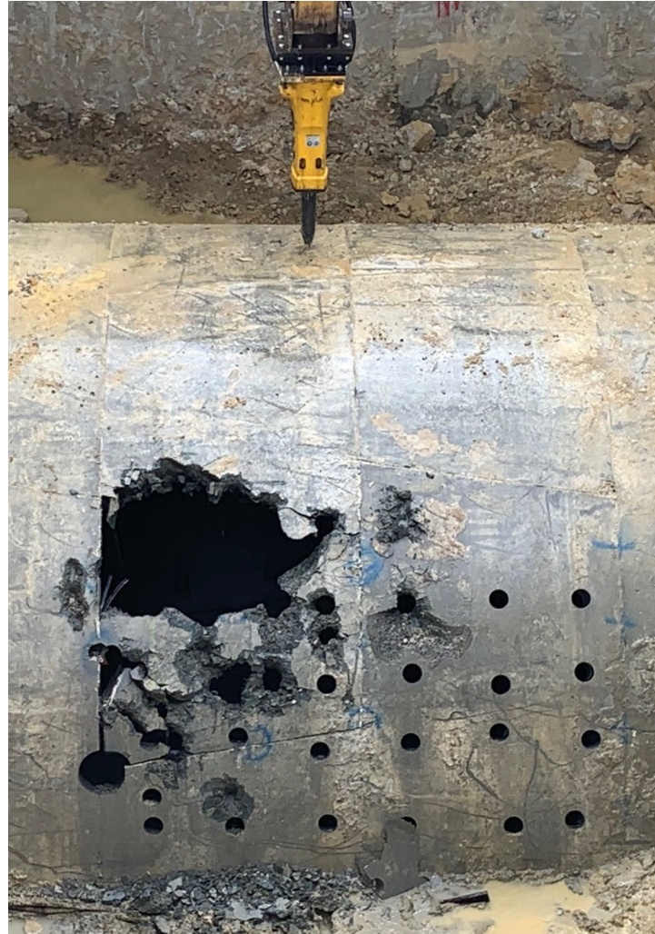
Sacrificial tunnel removal works
