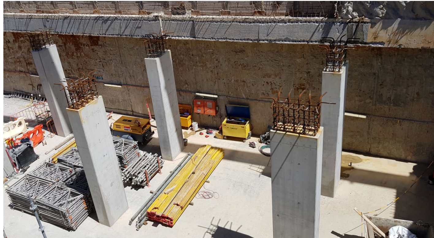
Internal columns poured in the Shrine entrance
