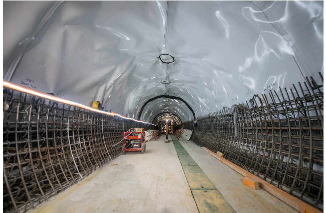
Partially constructed cross passage in Western Precinct, waterproofing membrane and steel fixing
