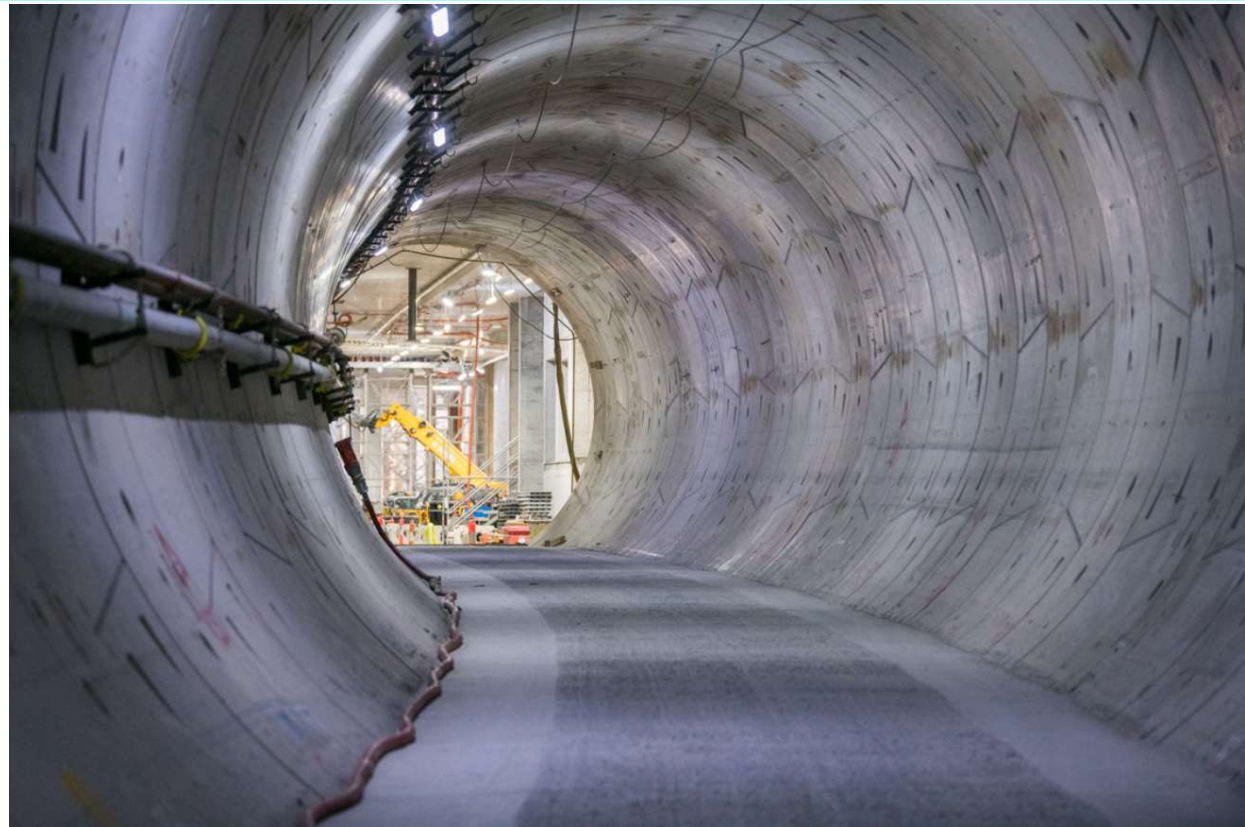
Completed invert concrete leading to Anzac Station
