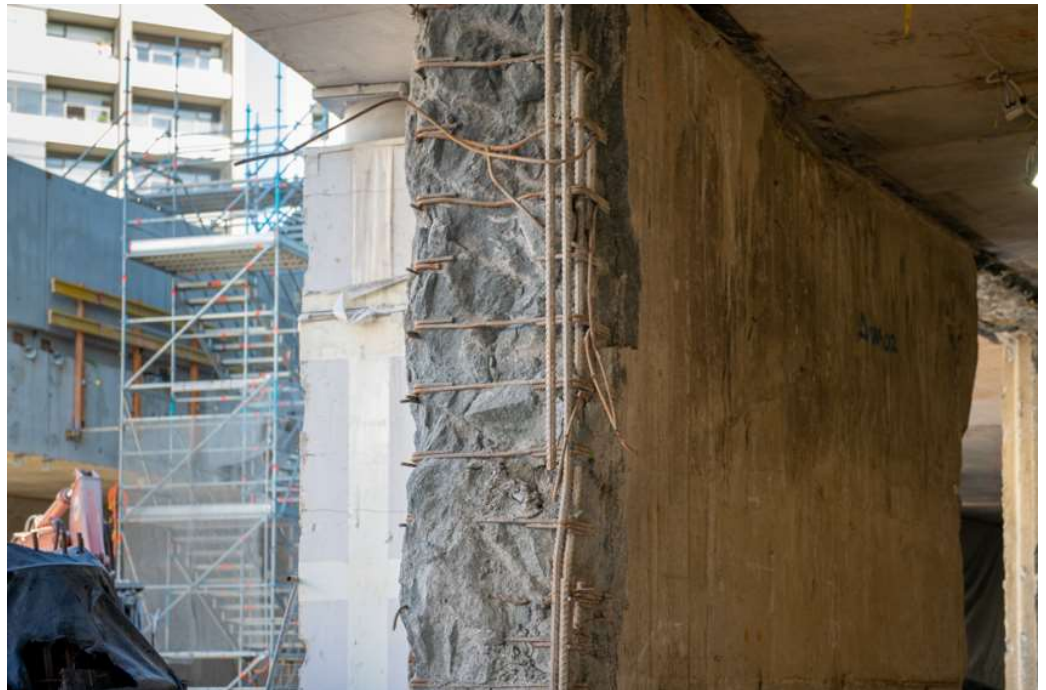
D-wall demolition – tram interchange to concourse
