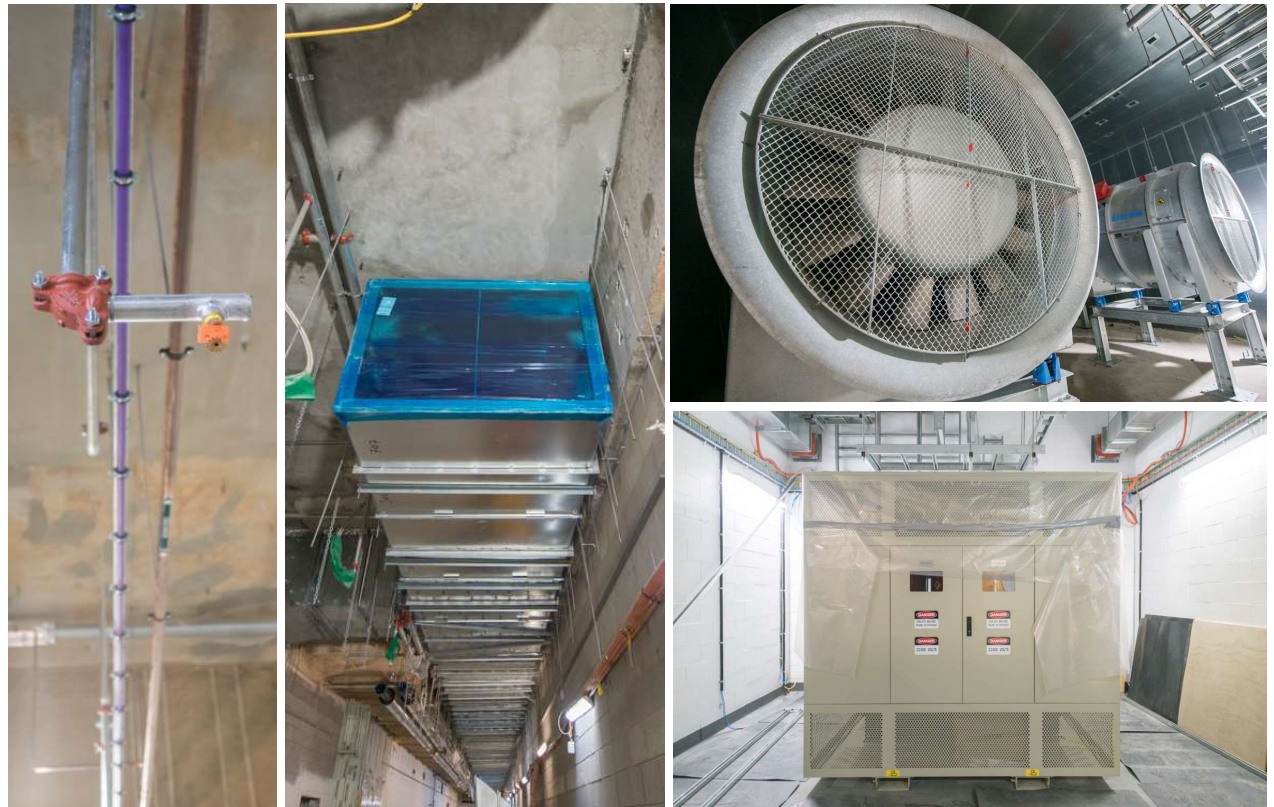
Wet fire services, ventilation, fan systems and power substation installation
