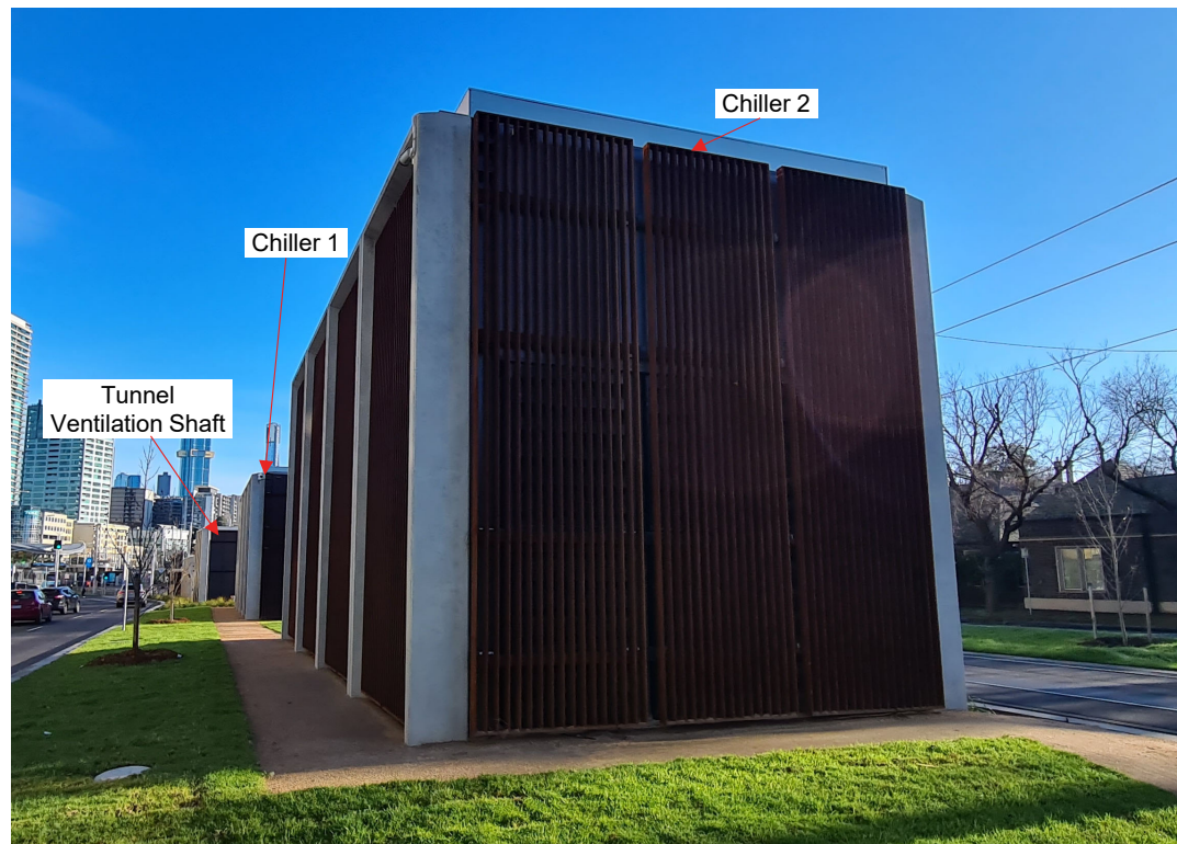
Acoustic insulation installation built around chillers
